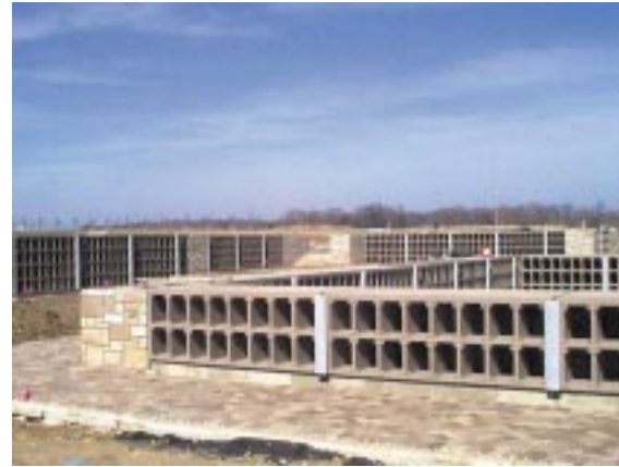
Columbaria under construction at Ohio Western Reserve National Cemetery.
